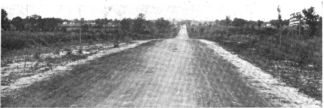
Experimental Stretch of Coal Tar Treated Road at Savannah, Ga., on Henry Street, Looking Westward into the Suburbs.
